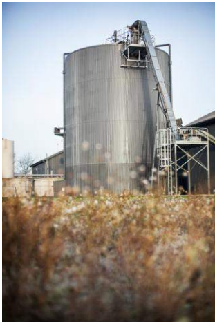
Fermenter and feed in system at Foulum Biogas Plant. Photo: Søren Tobberup, Aarhus Universitet
