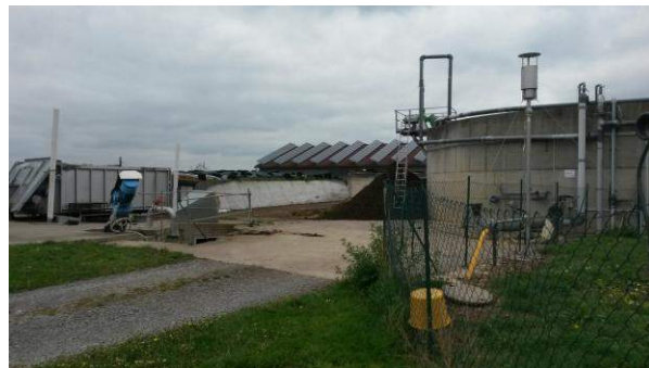
Residue storage tank with prior separation (right) as flare (right in the picture), fermenter belowground under the solid dispenser (left). Also shown: gas line, stirrer, condensate pit (right behind the yellow bucket)
