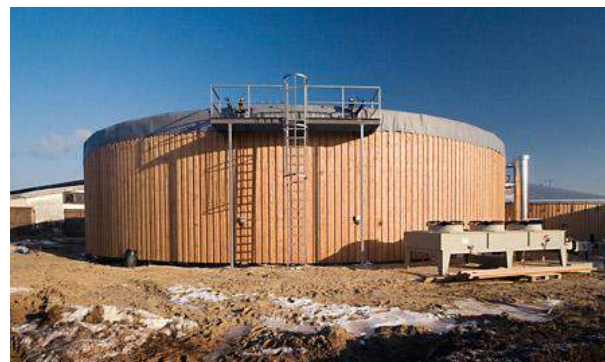
Biogas digester encased with wood for a better integration of the farm into the landscape.
